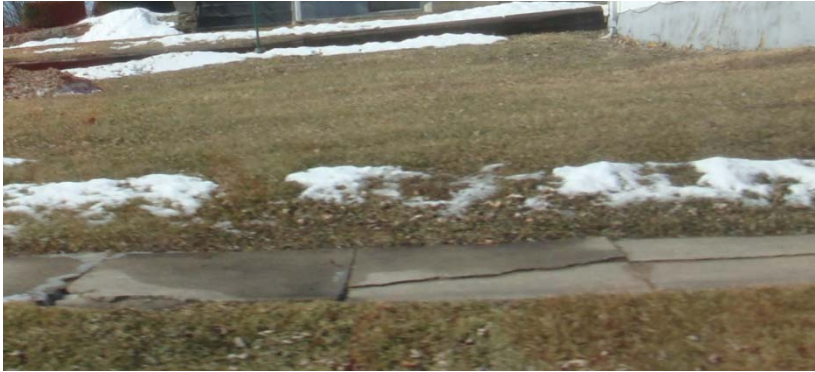
Figure 13: An example of a poor sidewalk observed in West Union
