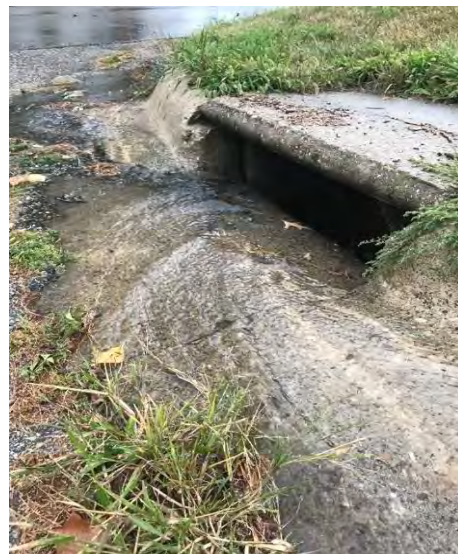
Common Stormwater inlet
