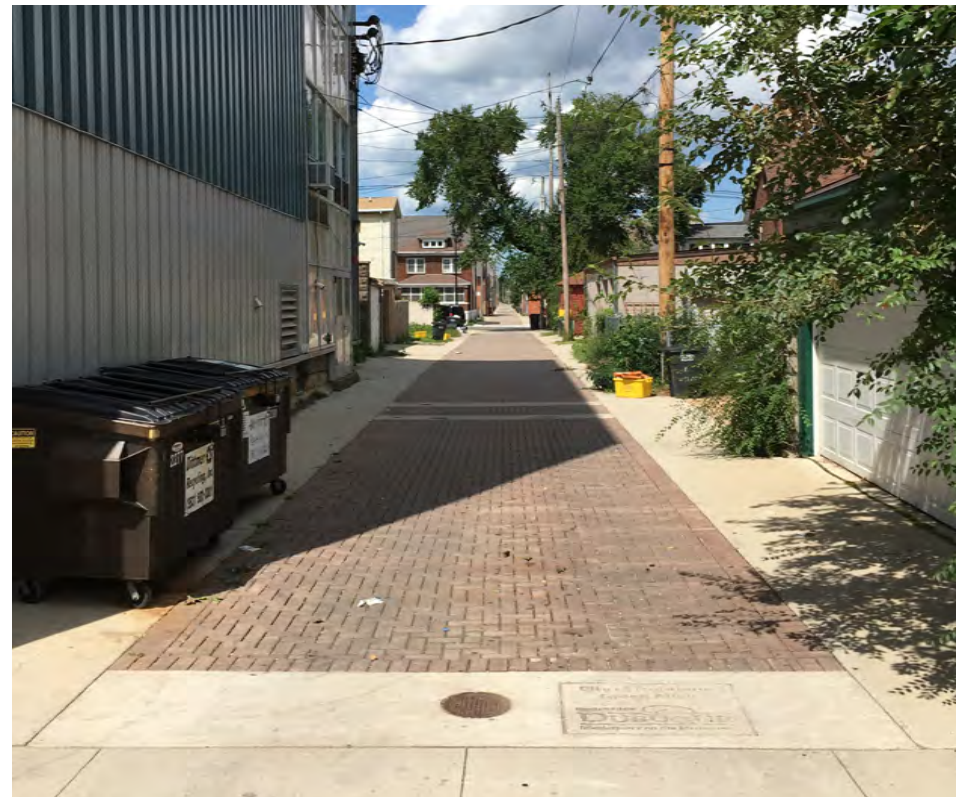
Part of Dubuque's extensive network of downtown "green alleys," with permeable pavers
