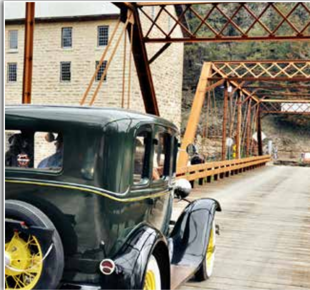
Motor Mill Bridge Reconstruction Project
