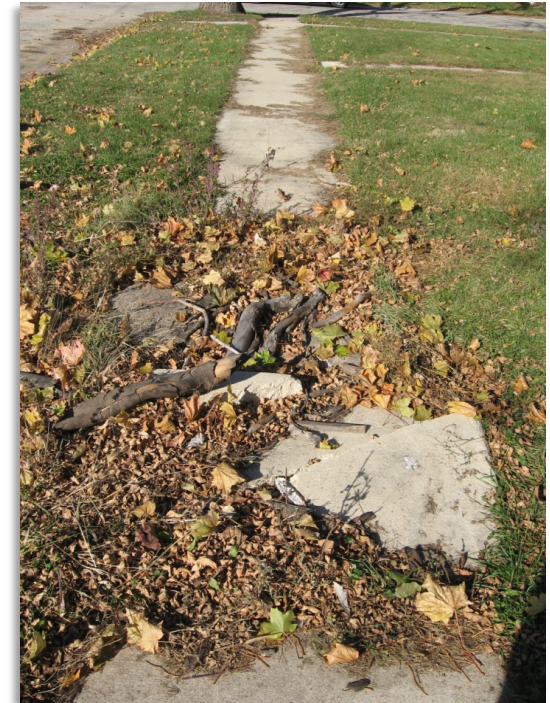
Sidewalks with large cracks, uneven slabs and rough surfaces can cause safety hazards for children walking and particularly biking to school.
